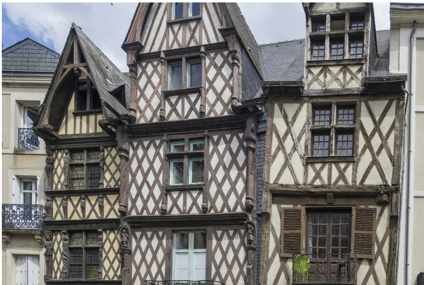
Original half-timbered houses still line a number of streets in Angers. Photo by Snap Wander on Unsplash
